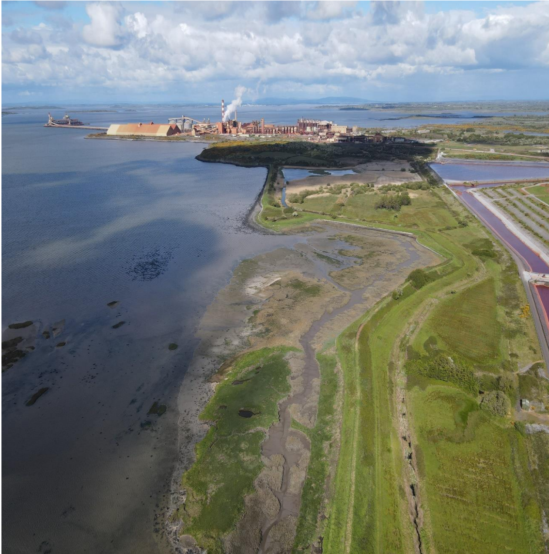
Figure 3. Photo of the lower Shannon estuary SPA along Aughinish shoreline.
